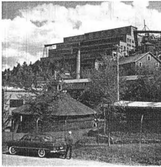
South Dakota is a major mining state. This is the Homestake Mine in town of Lead, largest gold mine in the Western Hemisphere
