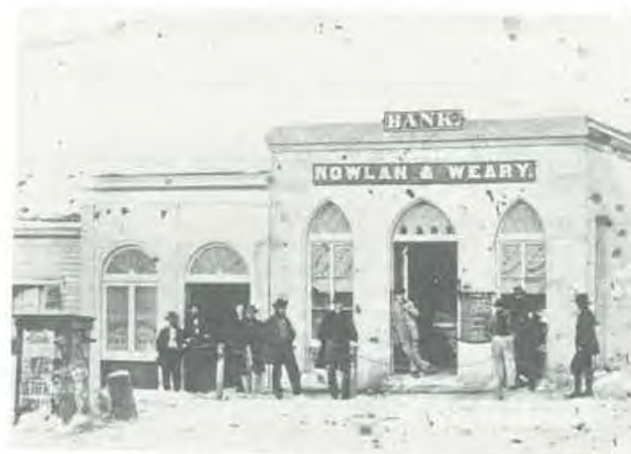
Nowlan and Weary Bank building in Virginia City, Montana Territory, 1866. Isaac I. Moore stands in door of executive offices at left. (Courtesy of Montana Historical Society.)
