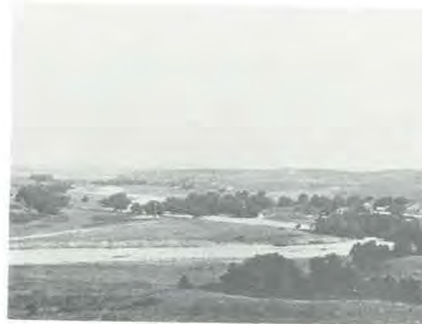
Ash Hollow. Wagon trains on the south side of the North Platte River moved through this defile. The Collins party passed north of the river (in background).
